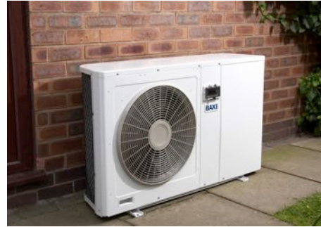
An Air Source Heat Pump (left) with an external unit, gathering heat from the surrounding air. A Ground Source Heat Pump (right) gathers heat from the ground via boreholes.
