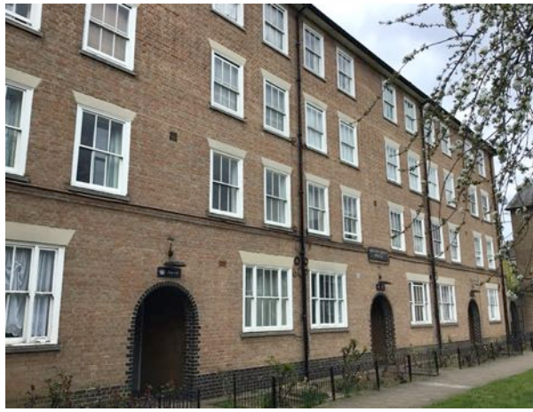
e.g. Barnersbury House, Holloway Estate
