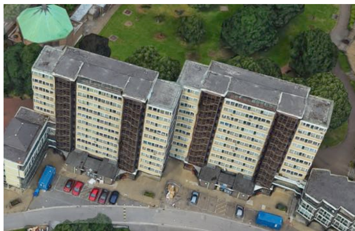
Colechurch House, Tovy House and Proctor House on the Avondale Square Estate appear to have large, unobstructed roof areas suitable for photovoltaic panel installation.
